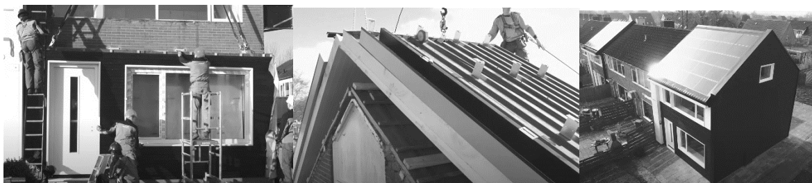
Figure 27 External insulation (wrap-it) (by VolkerWessels, 2015)
