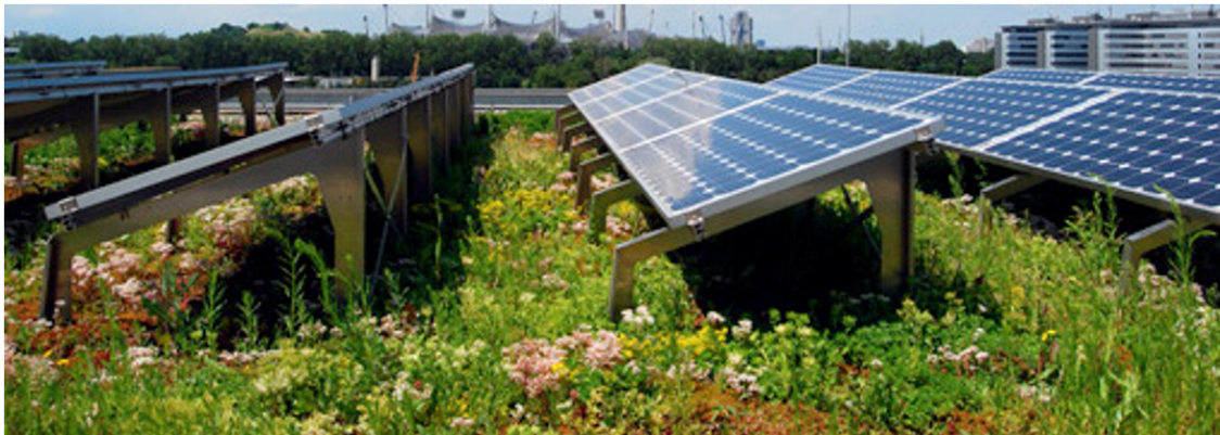
Figure 2.17: A Biosolar roof, photo obtained from (Renewable energy hub, 2020)
