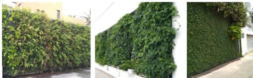
Figure 2.19: Living walls, indirect green facades, direct green facades (Galagoda et al., 2018)
