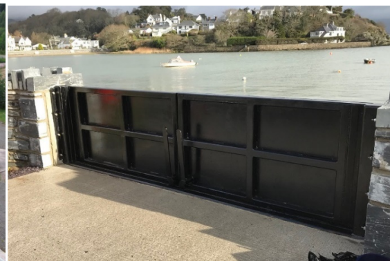
Figure 2.6: Flood gate in Buffalo (The flood company, 2020)
