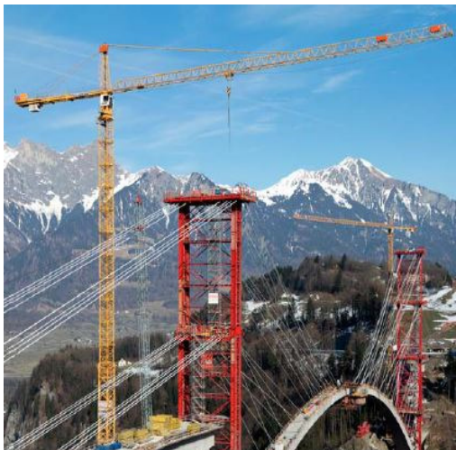
Figure 4. Top-slewing crane (Liebherr, 2016)
