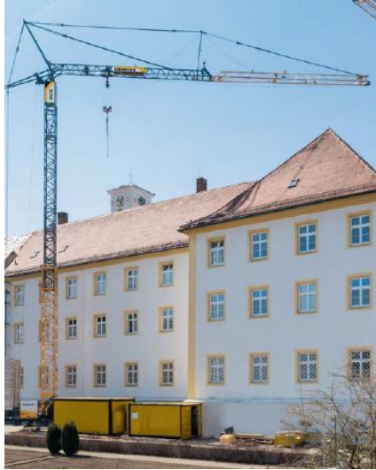
Figure 2. Fast erecting crane (Liebherr, 2016)
