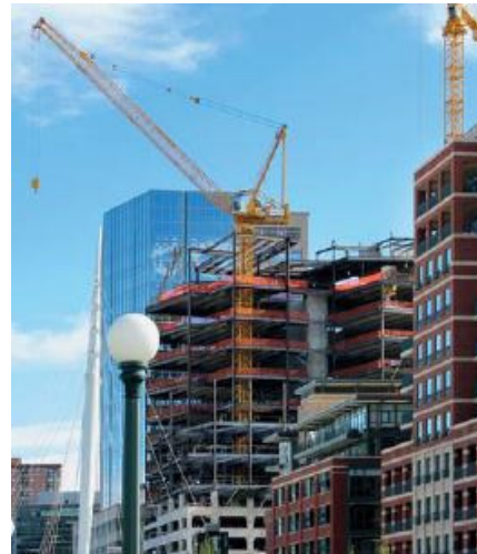
Figure 5. Luffing-jib crane (Liebherr, 2016)
