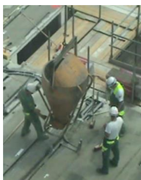
Figure 15. Fill concrete hollow-core slabs (Simons, 2016).
